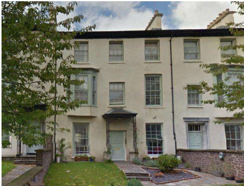
Georgian Terrace Townhouses - Clifton Place, Newport
