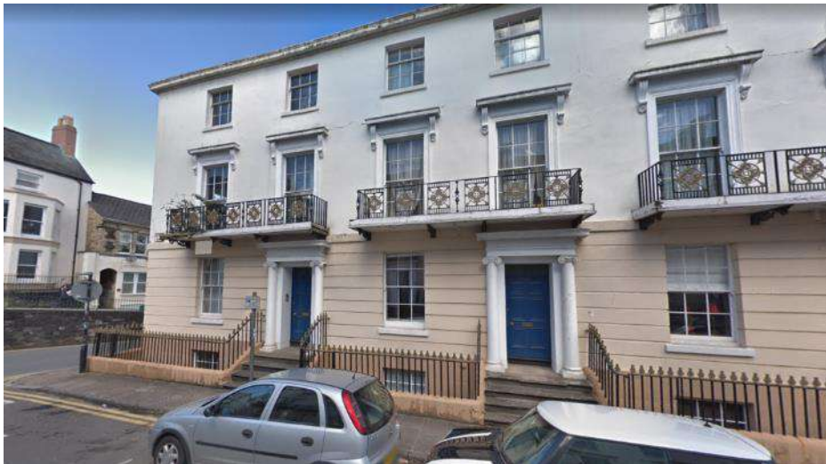
View of the existing residential dwellings on Victoria Place
