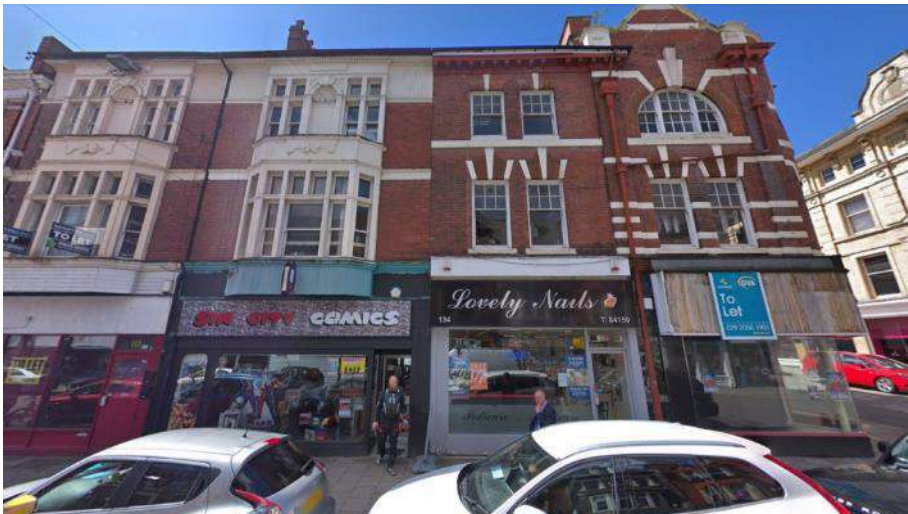
View of Front Elevation of existing properties - No's 133 - 135 Commercial Street
