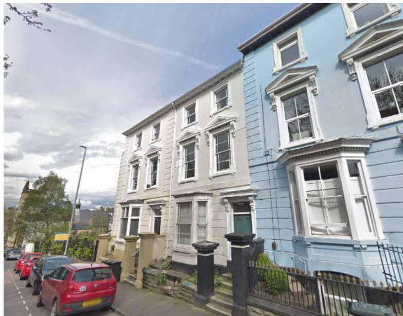
Georgian Terrace Townhouses - Clifton Place, Newport
