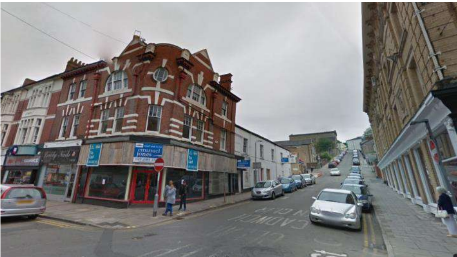
View of existing 135 Commercial Street looking up Hill Street
