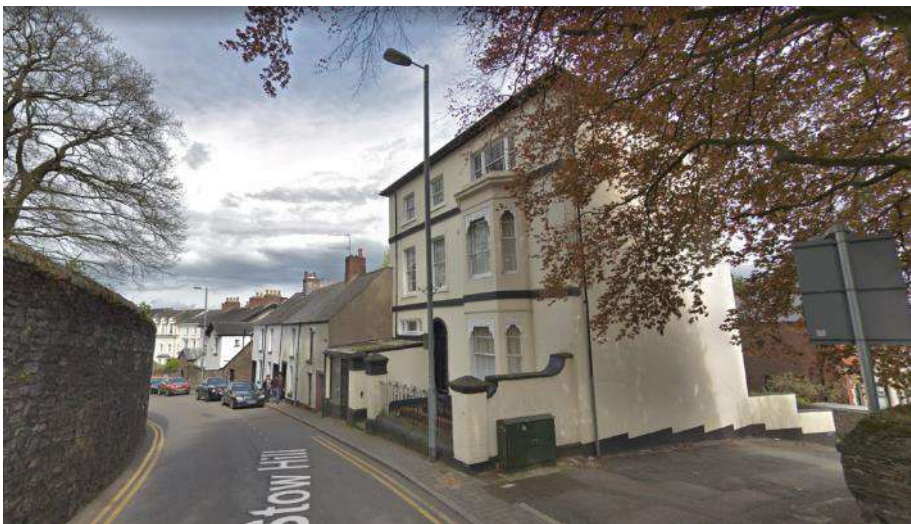
View heading East along Stow Hill towards Hill Street
