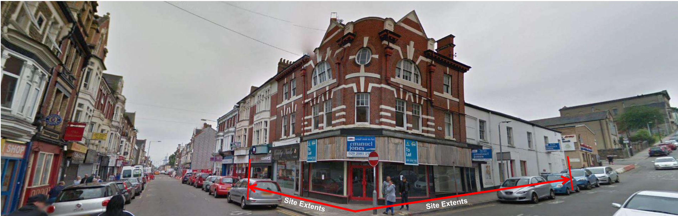
View from corner of Commercial showing existing South facing building facades
