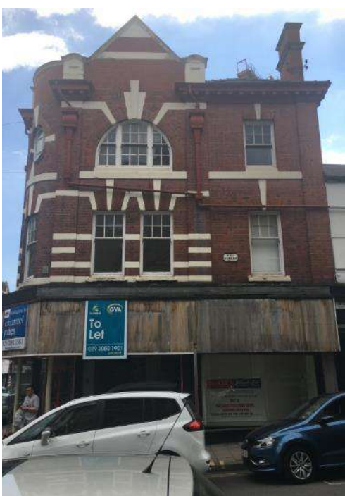
Northern Elevation of 134 -135 Commercial Street/ Hill Street
