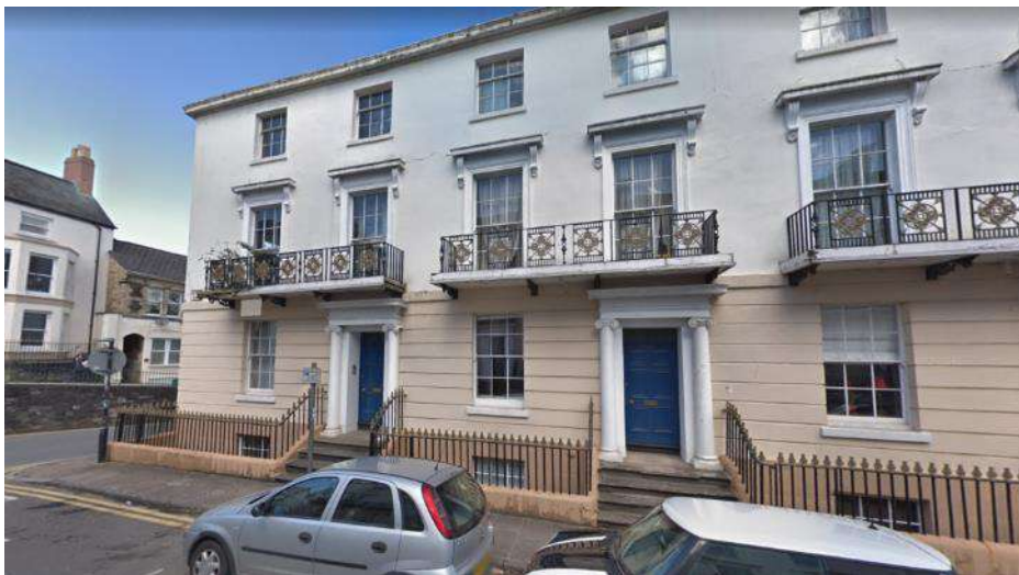
View of the existing residential Georgian Townhouses on Victoria Place
