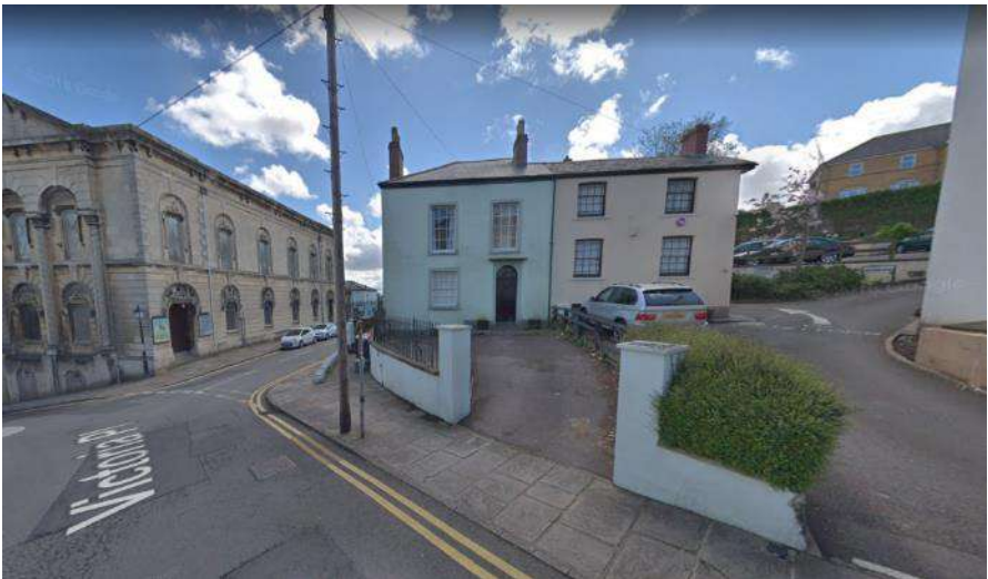
View of Victoria Place to the West of the Proposed Site
