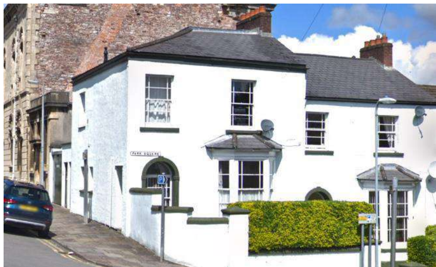
View of the existing residential dwellings on Park Square
