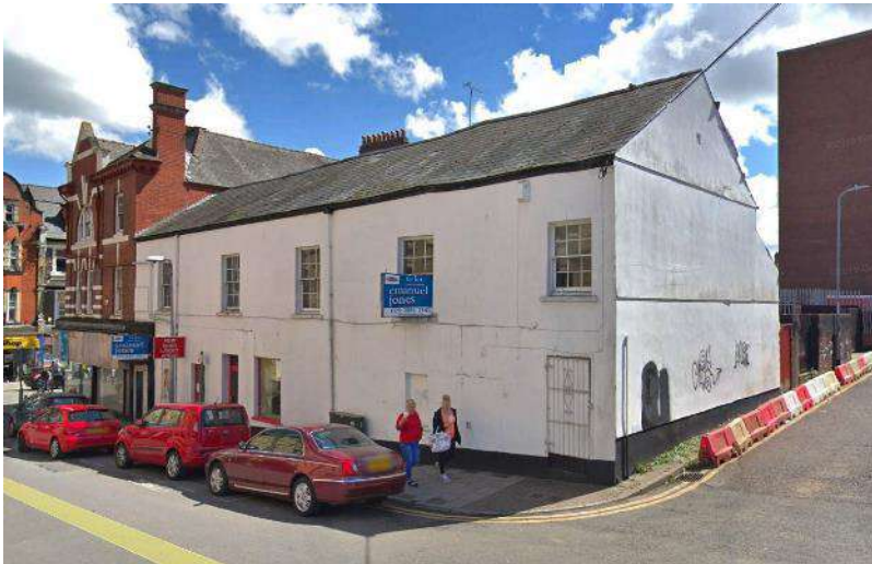
View looking South East at the existing rear annex on Hill Street
