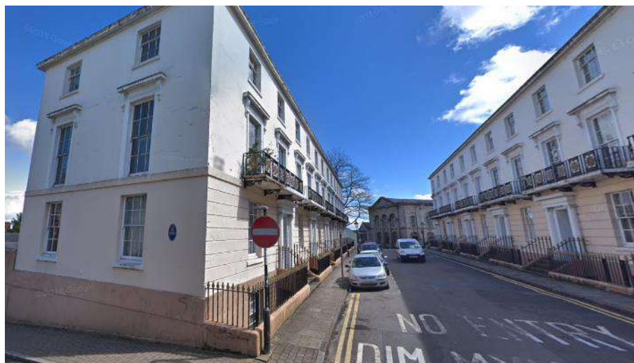
View of the existing Georgian Townhouses on Victoria Place
