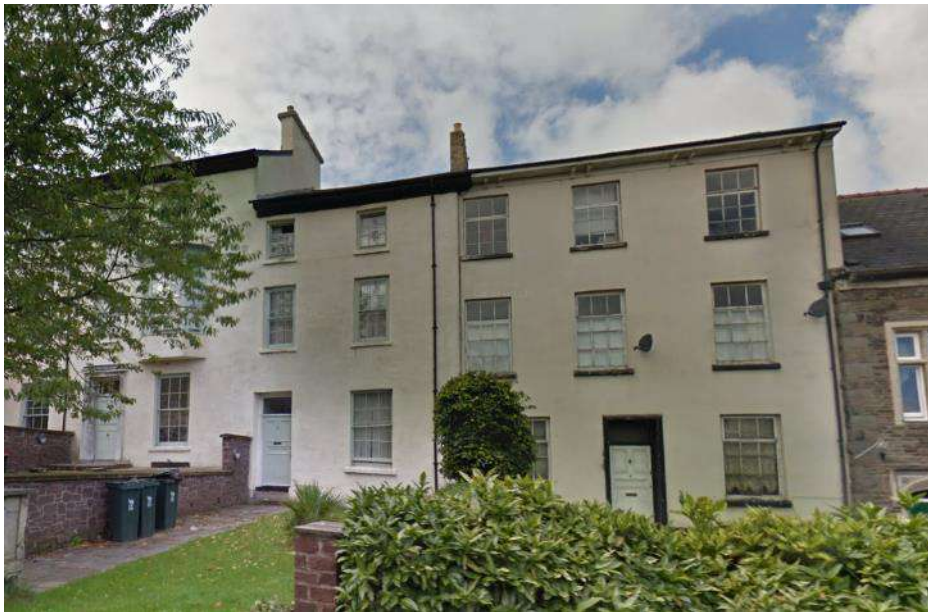
Georgian Terrace Townhouses - Clifton Place, Newport
