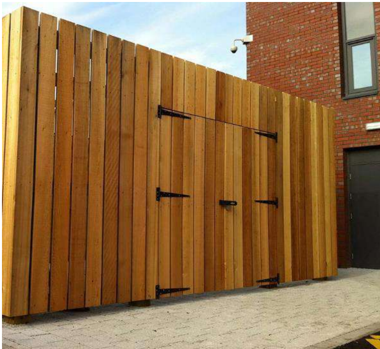
Rear Access - External Quality - Vertical tanalized timber enclosure - Painted & weather proofed
