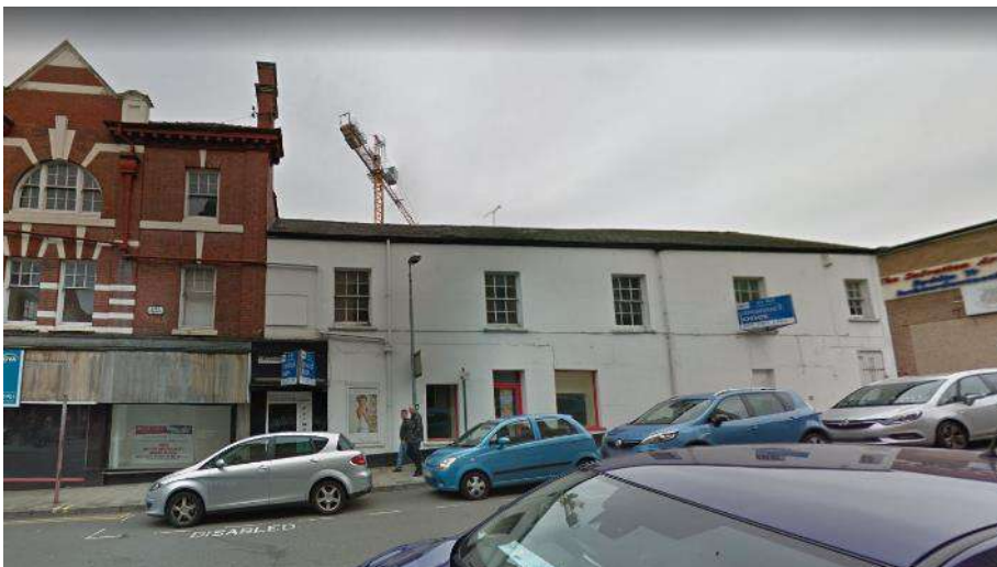
View looking South at the existing rear annex on Hill Street
