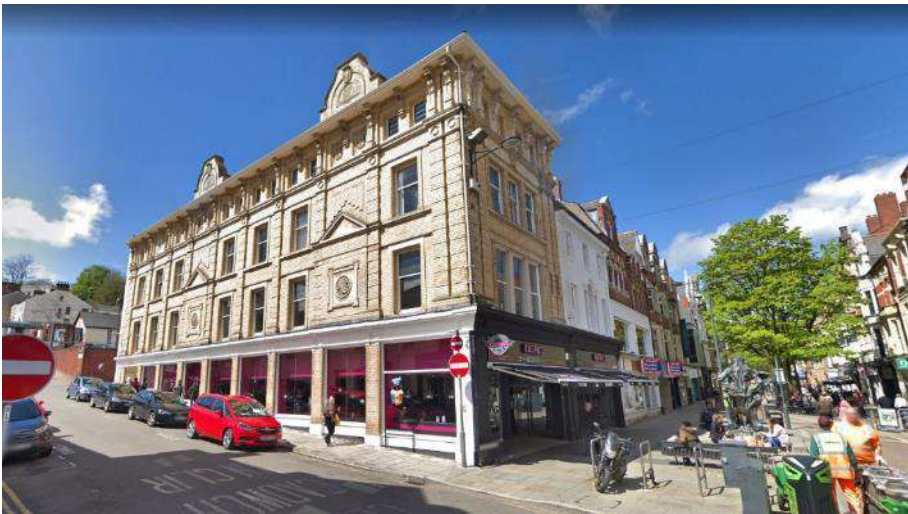
View of existing St David's House, positioned on the opposite corner of Commercial Street
