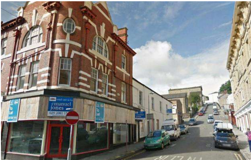
View of existing 135 Commercial Street looking up Hill Street
