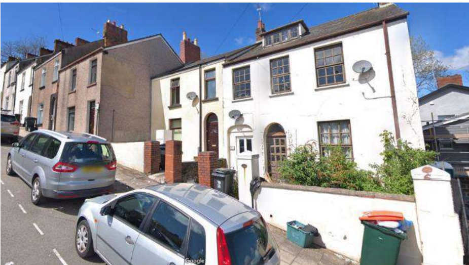
View of closest existing residential dwellings on Hill Street
