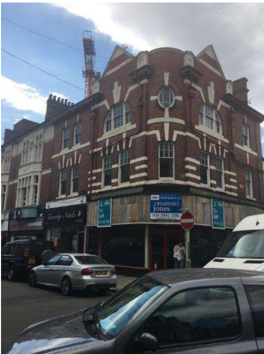
Corner Elevation of 134 -135 Commercial Street
