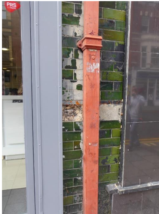
Fig 10 Evidence of glazed tile pub frontage to former Tradesmen's Arms
