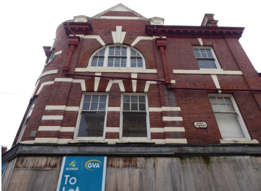
Fig 8 Hill Street elevation of former Tradesmen's Arms
