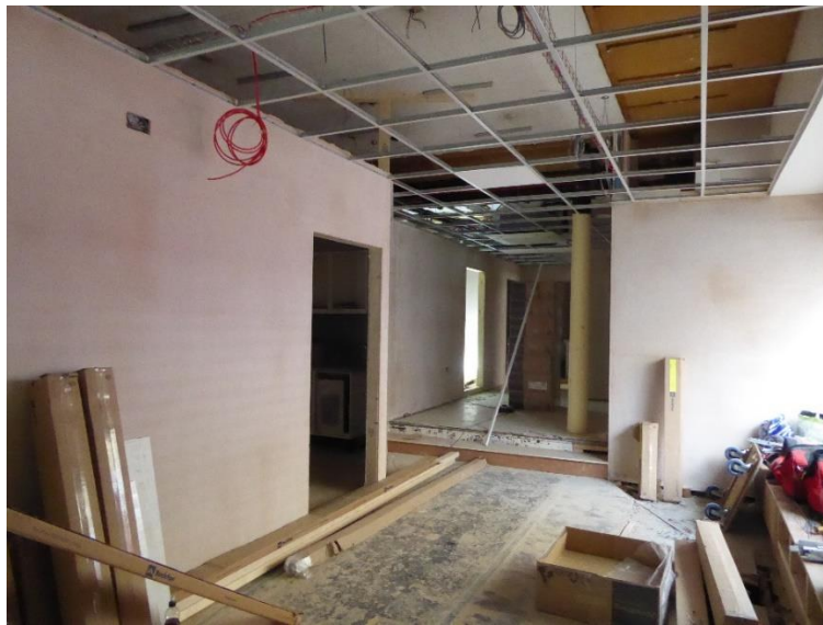
Fig 19 altered ground floor to No 135, the former Tradesmen's Arms
