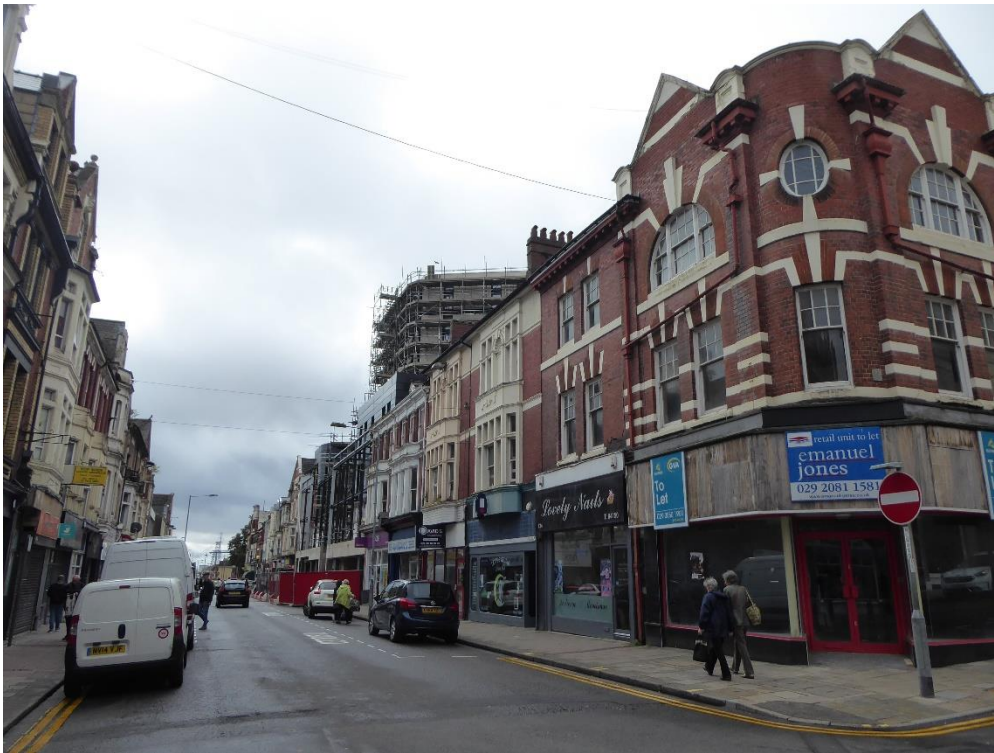
Fig 20 view south along Commercial Street with Nos 133-135 to the right
