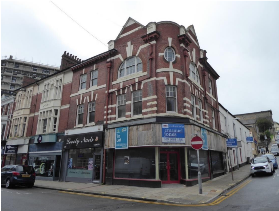
Fig 7 View from junction of Commercial Street and Hill Street
