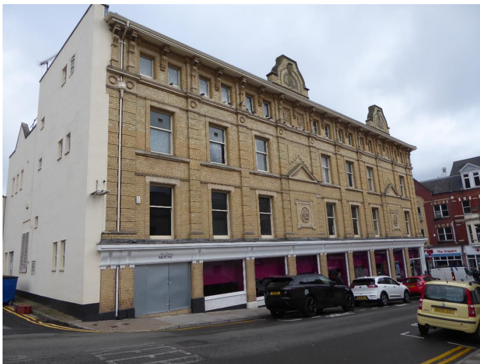
Fig 25 Hill St elevation of No 137 Commercial St opposite the proposed development site
