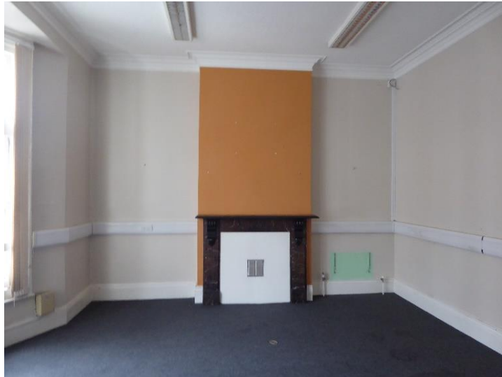
Fig 15 Interior view of 1 st floor bay-window room to No 133 retaining cornice and fireplace
