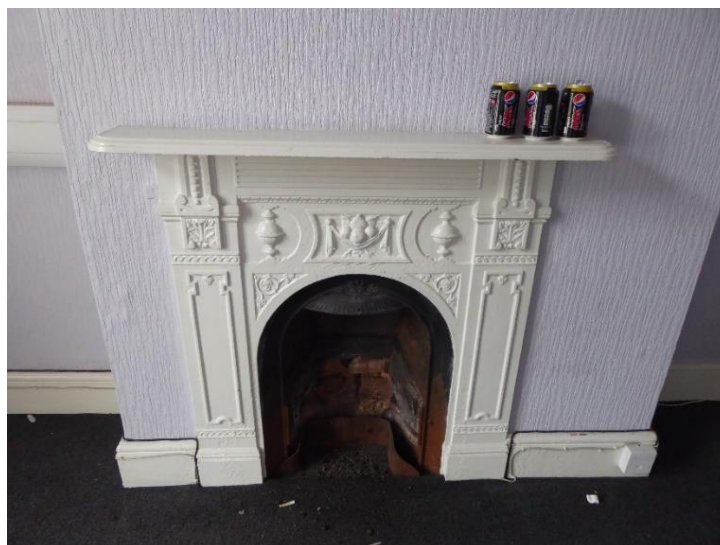
Fig 16 Surviving fireplace to 2nd floor of No 133
