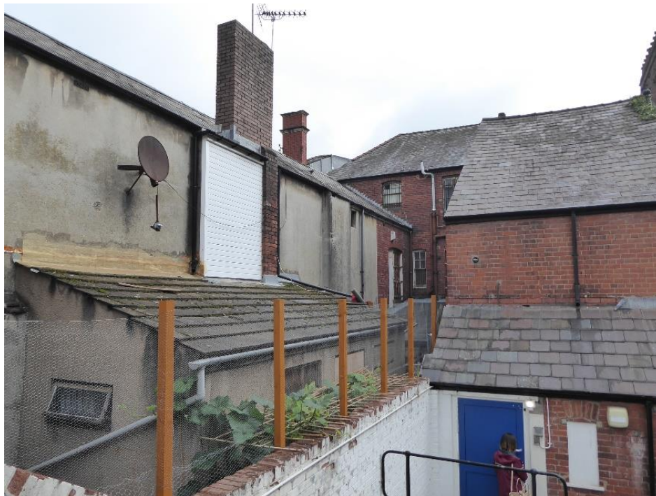
Fig 12 Rear elevations showing rear of Hill Street range to the left
