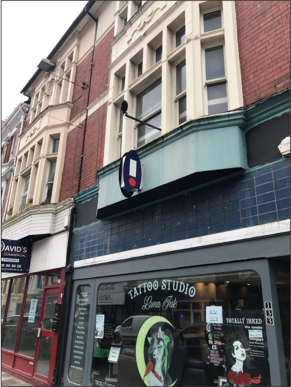
Figure 2 – View of Equipment Location, Front Elevation
